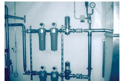
Compressed air systems: Monitor drier to avoid damage caused by humidity
